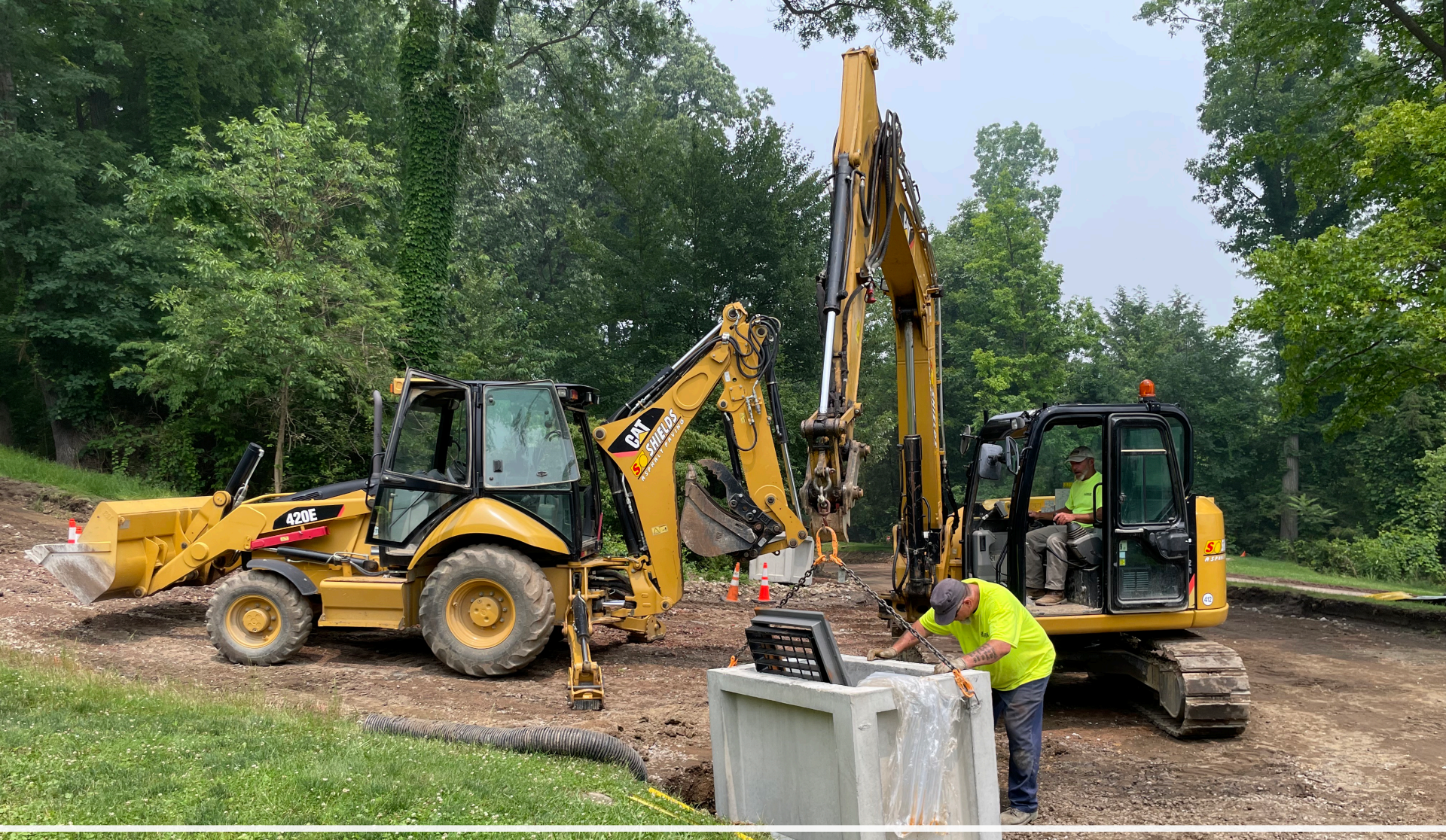
New storm drains
